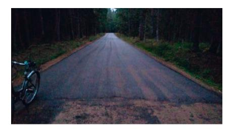
**Fig. 26:** Previously forest ground road being upgraded with a bituminous layer
